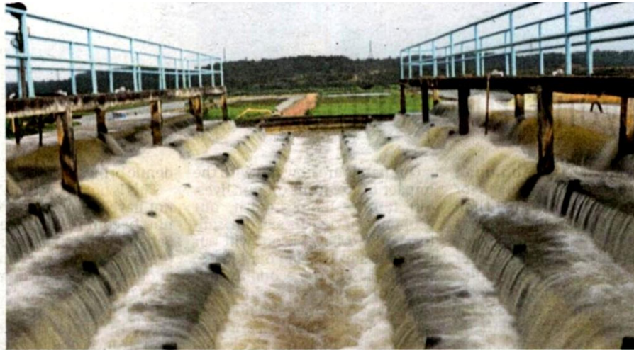
Phase 1 of the Sungai Selangor Water Treatment Plant. Laws and enactments are being strengthened to protect this vital resource. PIC BY SHAHMI IMRAN
